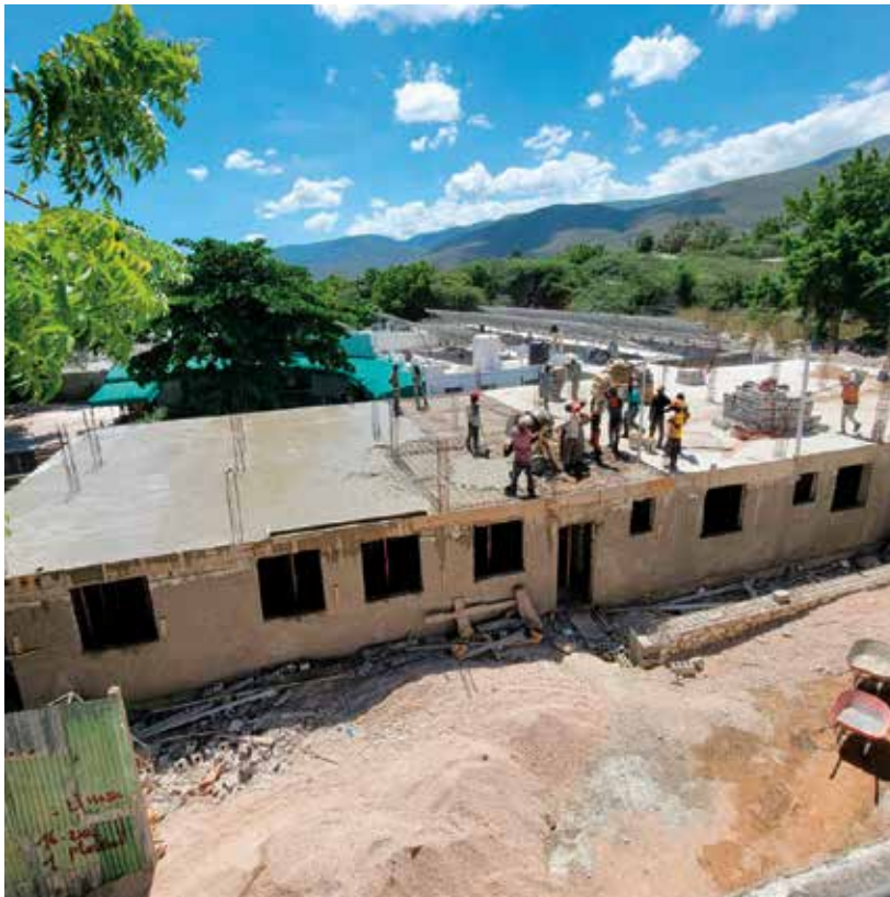
Construction of the maternity center will be complete this year.
