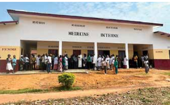
The new internal medicine building at the St. Vincent the Servant General Reference Hospital, run by the Daughters of Charity
