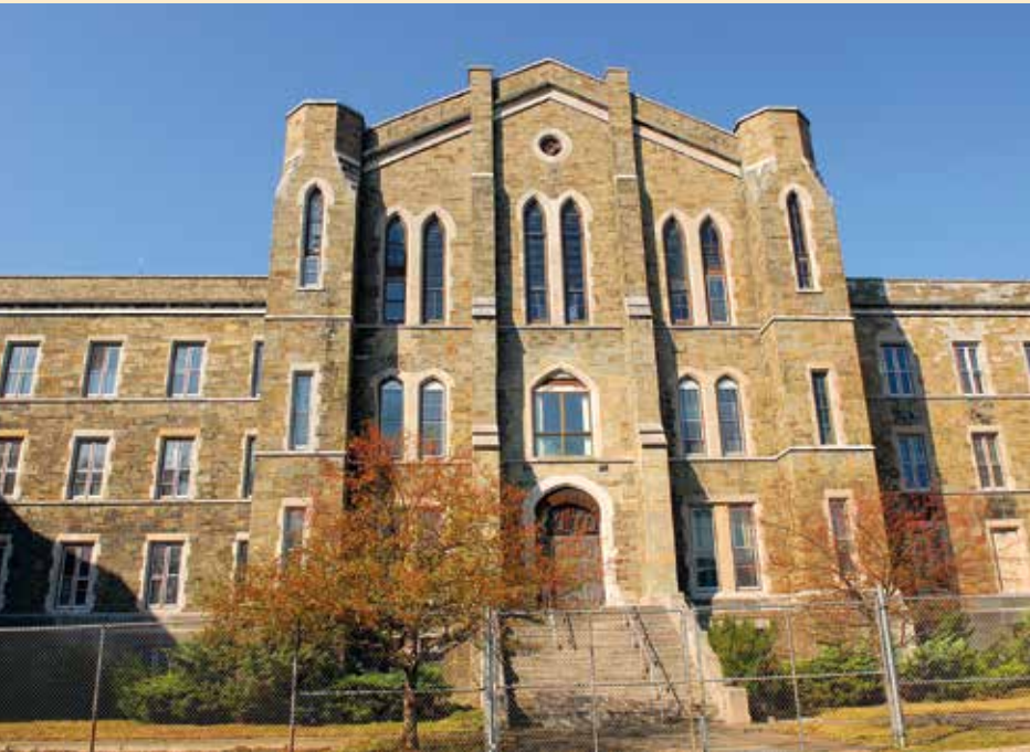
A former state asylum building in Binghamton will become home to Upstate's Binghamton campus and clinical skills assessment center.
