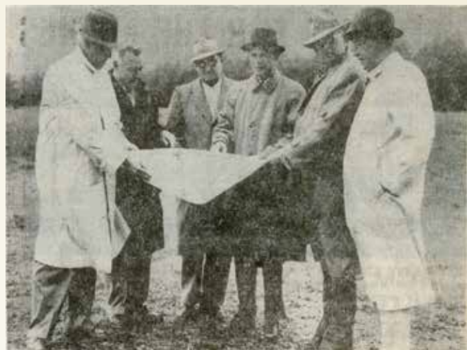
Harry King, architect, Dr. Albert Snoko, consultant, George Cooper and David Jasper, building committee members, and Thad Collum and Carl Maar, hospital fundraisers, look over the tract of Onondaga County Sanatorium land as the probable site for the new Community Hospital on May 4, 1958.
